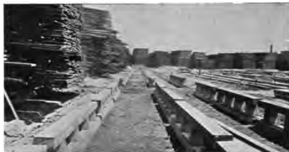
Fig. 7.* Concrete Lumber Supports, to prevent contact with earth affected by dry rot.
